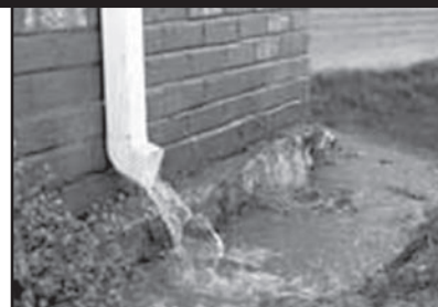
DIRECT RAINWATER AT LEAST 4 FEET AWAY FROM FOUNDATION
